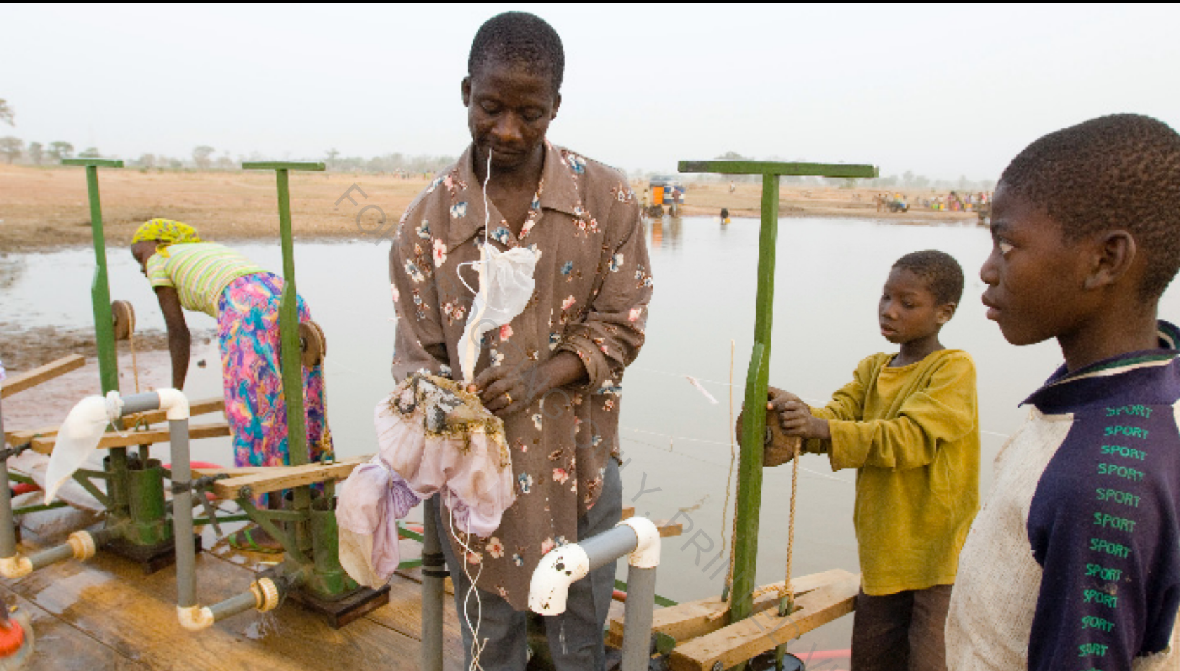
Dam guard Alhassen Alhassen changes the filter on a SOKA water pump. Paid for his labors with a bicycle to ride to work each day, his job is to prevent anyone with an emerging Guinea worm from stepping into the dam.
